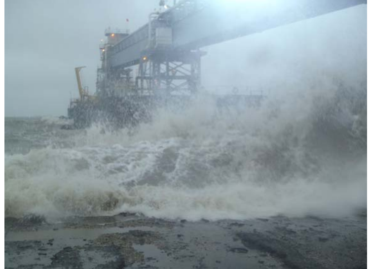
Waves crashing into the P10 gallery (covered conveyor belt) during the storm on August 25, 2012 at the port site.
